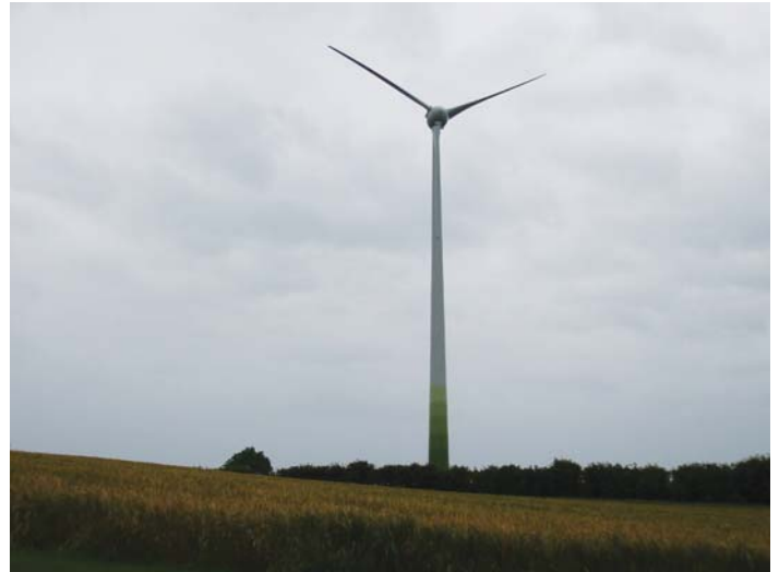
The turbine at Braidenhill Farm, near Glasgow, Scotland.
